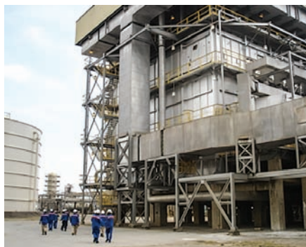
FIG. 10. Plant operators and inspectors approach a reformer for hands-on single-point infrared pyrometer training.
