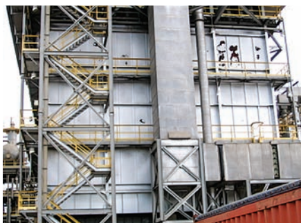
FIG. 5. Low-emissivity silver paint common on reformers.
